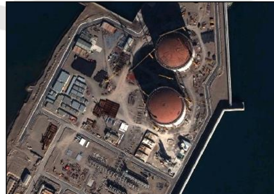
Monitoring of construction works of a regasification facility.
